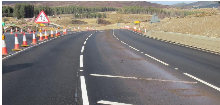
Photo 2: Hatching missing from lane past the junction
