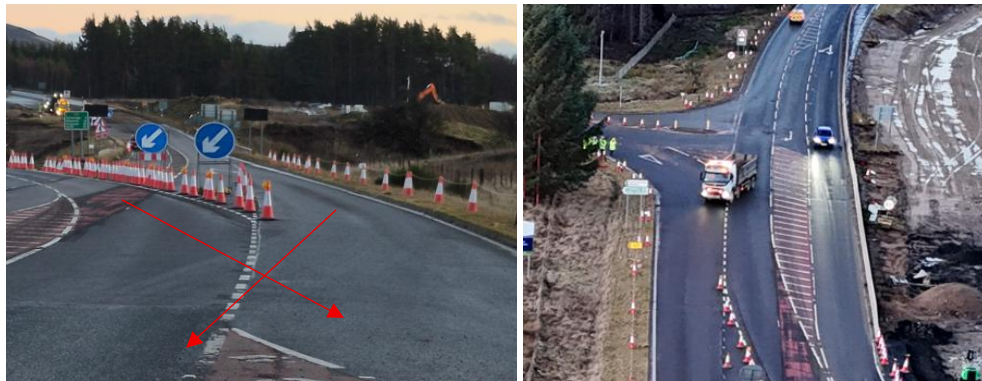
Figure 1: Works Access Exit.
