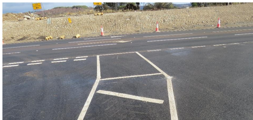
Photo 3: Marked separation island at the junction
